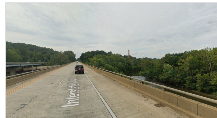
View west from the bridge over the Rivanna River.
